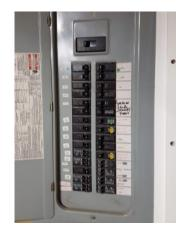
The 240VAC circuits are connected to an intermittent panel. These circuits operate as normal, on loss of utility power they will only operate with the generator. A very small Mi-Grid system can power a large house or business with little or no inconvenience and saving significant capital costs.
